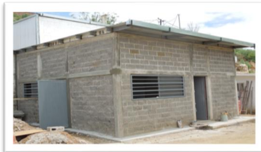
New Electrical Substation
