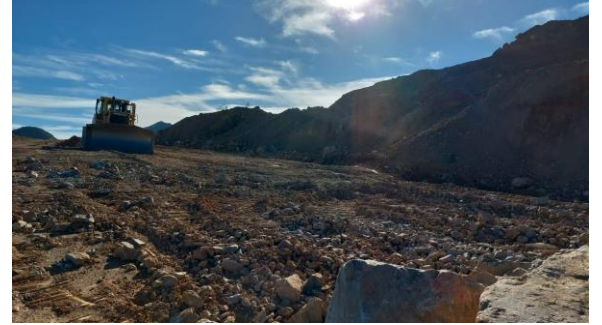
Ground pads ready at the Avino property
