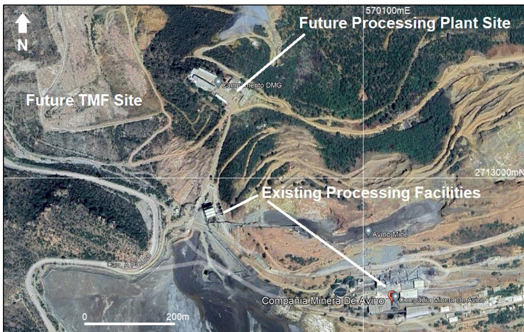
Figure 18-1: Existing Road Network at Site (Tetra Tech, 2023)
