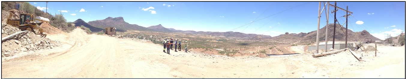
Figure 18-2: Typical Internal Access Road at Site, Panoramic View (Tetra Tech, 2023)
