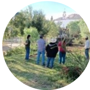
Cleared brush from outside of the schools in San Jose de Avino
