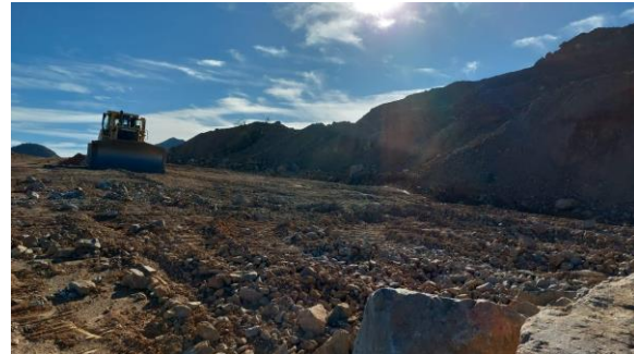
Ground pads ready at the Avino property
